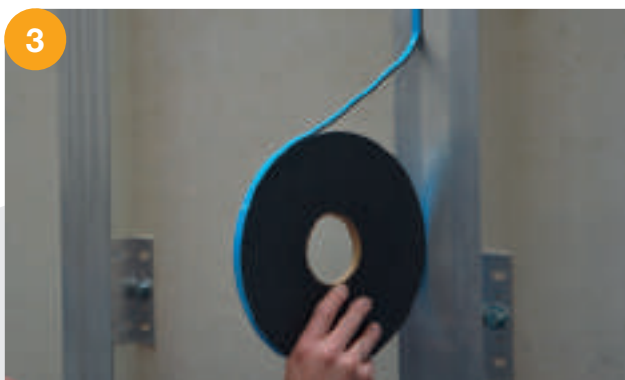
Klebeband anbringen
